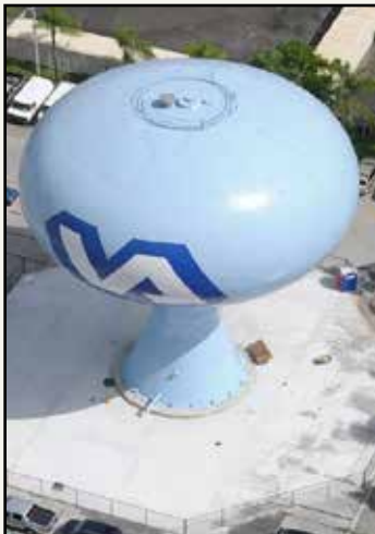
Design-Build 1-Million Gallon Elevated Storage Water Tank, Miami VA
