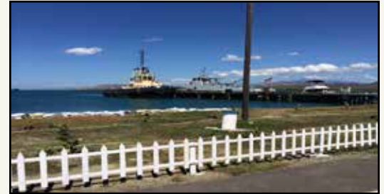
Renovations for FY14 Tradewinds Exercise Las Calderas Naval Base, Dominican Republic
