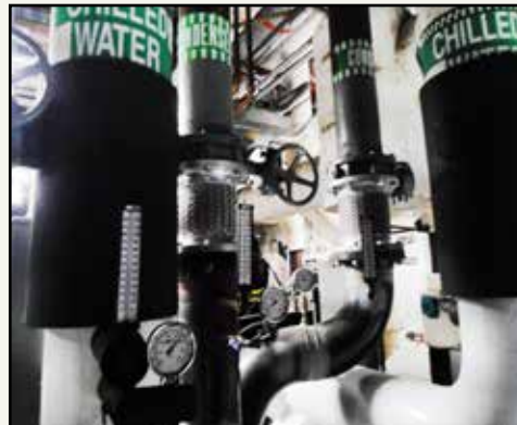
Replace Two Centrifugal Chiller Units NSA Orlando
